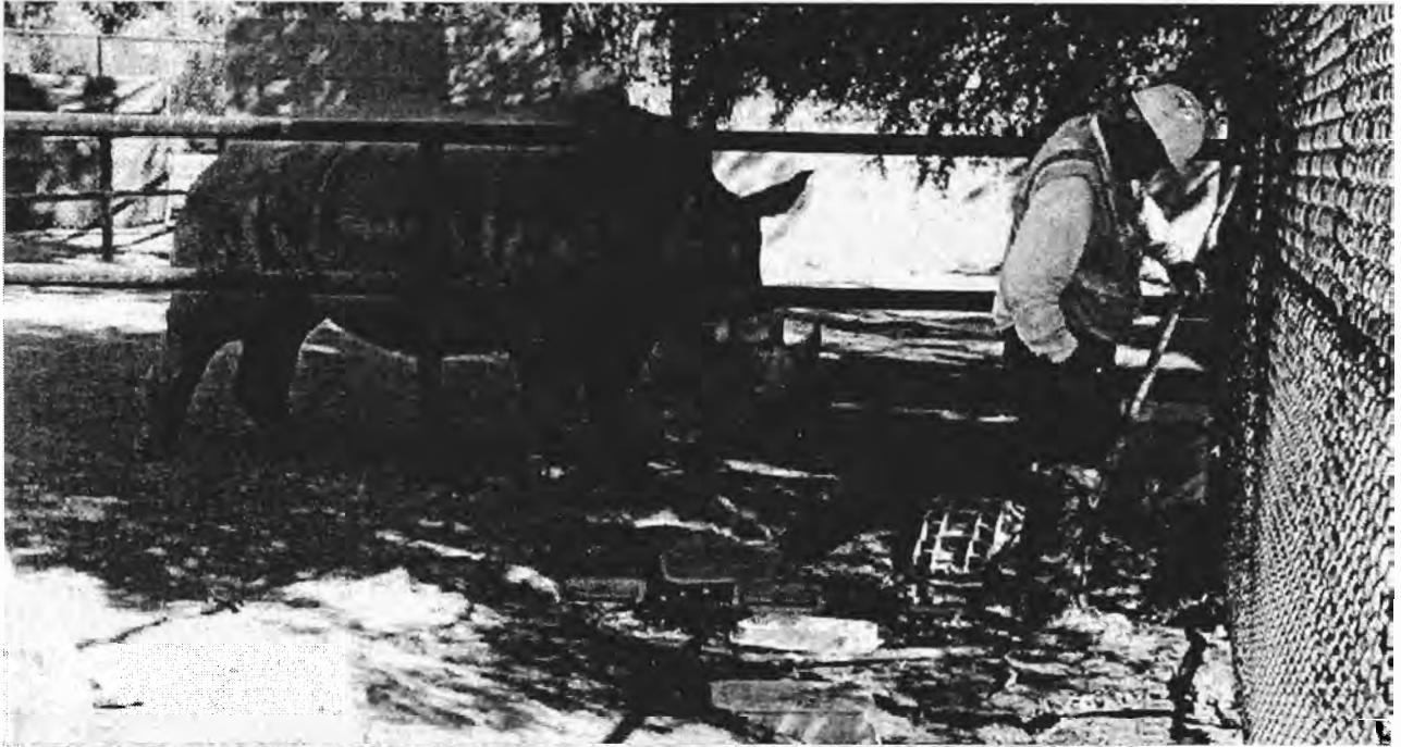
A worker checks recycled water infrastructure near one of the new resident rhinos at the African Adventure exhibit at the Fresno Chaffee Zoo, which opens tomorrow.
